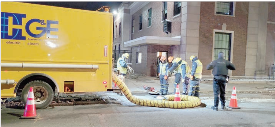
An explosion underground blew manhole covers off near a building in mid-January.
