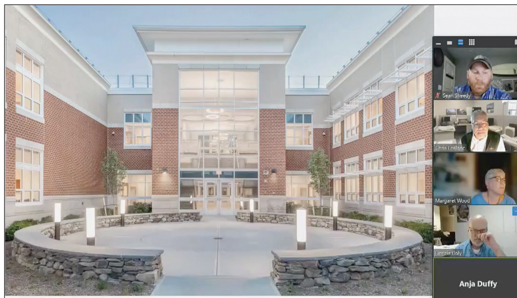
Senior Associate from the Mount Vernon Group Architects Chris LeBlanc walks through the layout of the outdoor classroom area in the courtyard.
