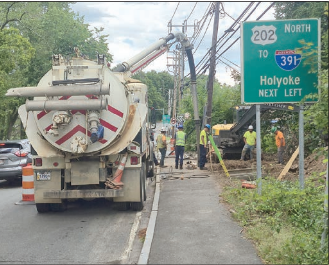
Turley Photos by Brendan Rooney Crews on site as they remove and drain the water.
