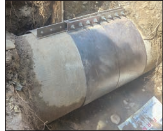
The water main transmission line that was close to being fixed late this week.
